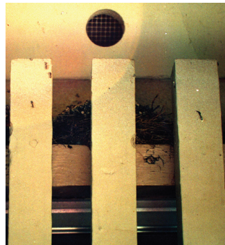
A typical bird's nest on a louver in the base housing area.
